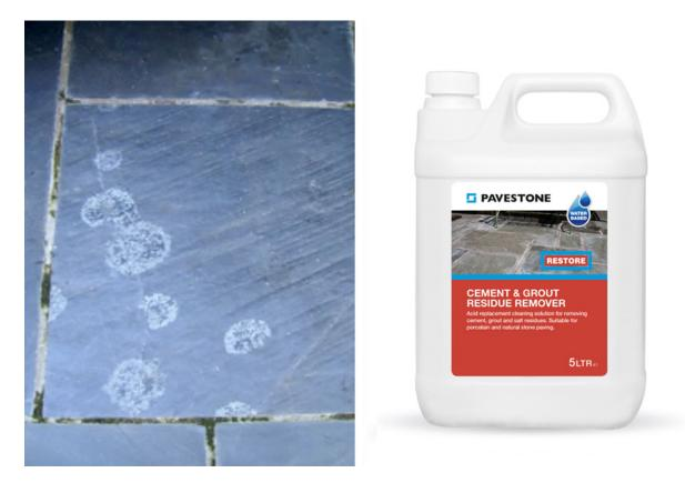
Slate contains calcites, deposits of this mineral at the surface of the stone can sometimes cause white spots or blooms with a flaky appearance to form on the surface of the paving.
