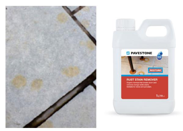
Ferrous sulphates contained in many common garden fertilisers can leave rust coloured spots and stains on paving. This is often seen where a patio meets a lawn or flower bed. Fertiliser manufacturers advise that paving should be covered before applying.
