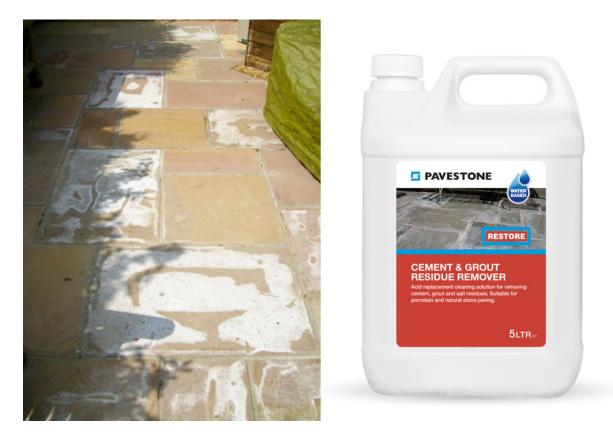
Efflorescence is caused by lime in the cement used to bed paving is absorbed and drawn to the surface. This is a natural phenomenon that can happen at any time and causes unsightly blooms and often occurs when paving has been laid incorrectly, on spots of mortar rather than a full bed.
